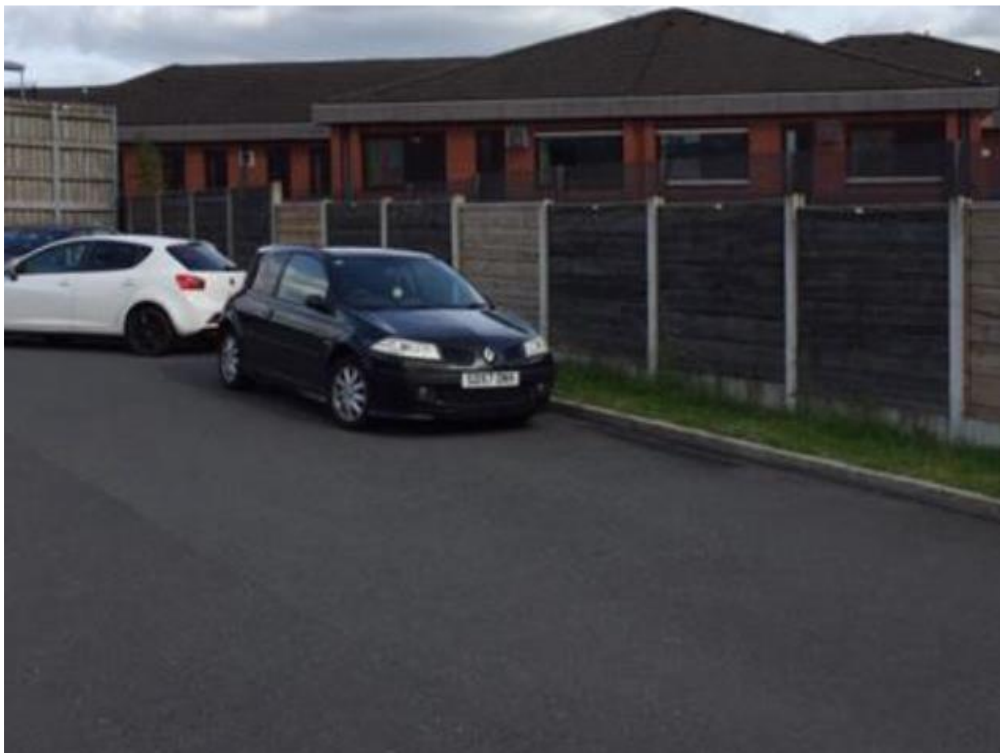
Photo 2 – view of north western corner of the existing building
